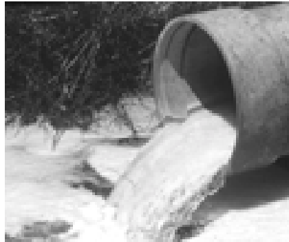
A direct discharge from a pipe is point source pollution and can usually be traced and identified.
