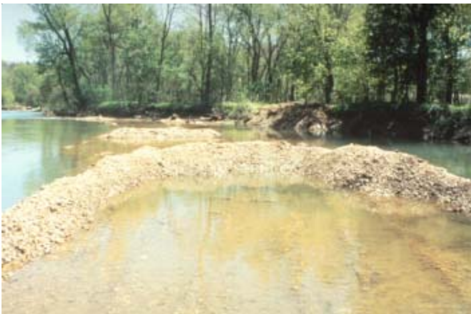
Removing gravel from below the water line can increase stream instability and destroy aquatic habitats.
