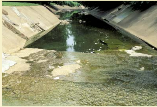
Channelized and armored streams with heavy stormwater runoff are unstable and transfer problems downstream. Channelization and armoring will lead to eroding streambanks above and below the channelized reach.
